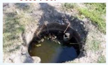
underground holding tank (sealed at the bottom) or a soak pit (not sealed at the bottom).
